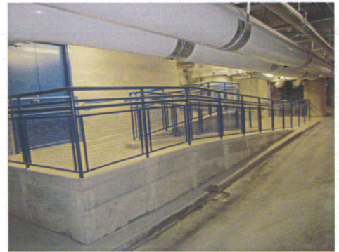
The new City Hall staff pedestrian ramp
