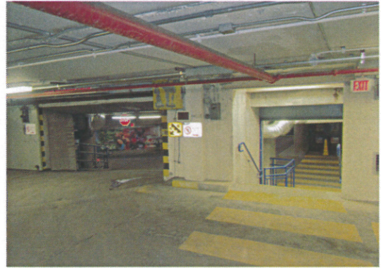
The new stairs and ramp make it safer and easier to access City Hall
